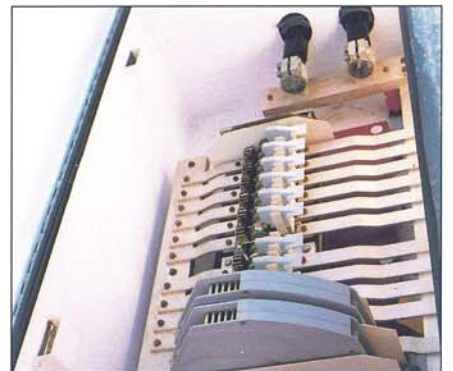
2500 Amp Load Break Switch
